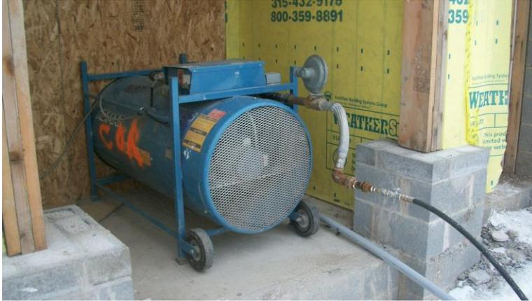
**Improperly Installed Temporary Heating Unit. This unit was installed not in accordance with the manufacturers guidelines (inadequate clearances to combustible building components) and posed an immediate fire hazard to this \$16 million wood frame apartment complex.**
